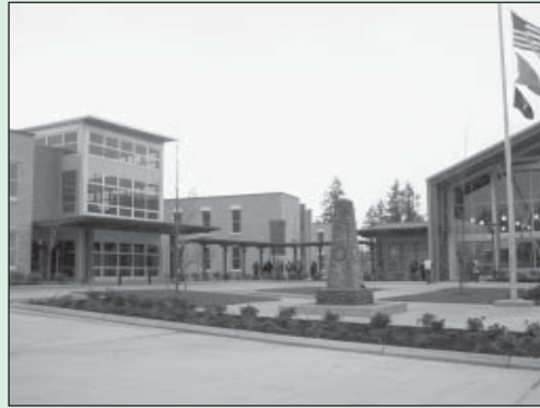
The new state-of-the-art facility at the Washington Veterans Home is located on a 31-acre bluff across Sinclair Inlet from the Bremerton Shipyard. This Home serves over 300 residents needing both long-term nursing and assisted-living care.
