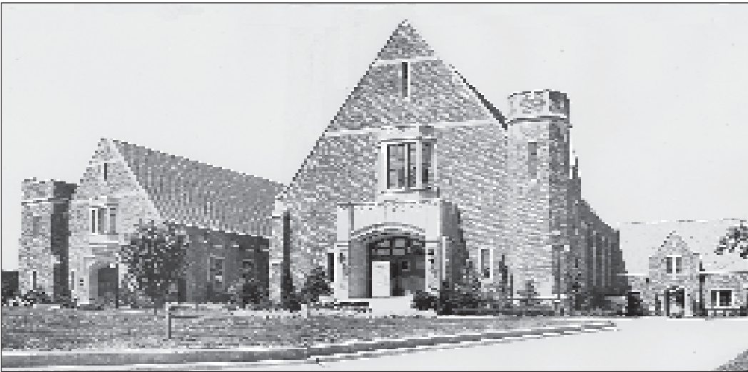
Auditorium / Dining Hall
