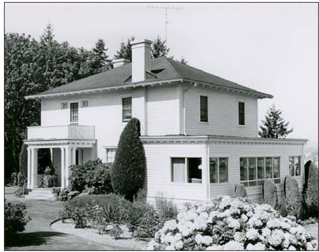
The Superintendent's Home, is still used by the current superintendent.
