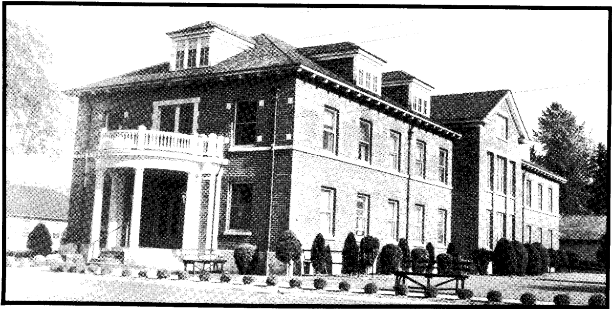
Roosevelt Barracks (west wing).
