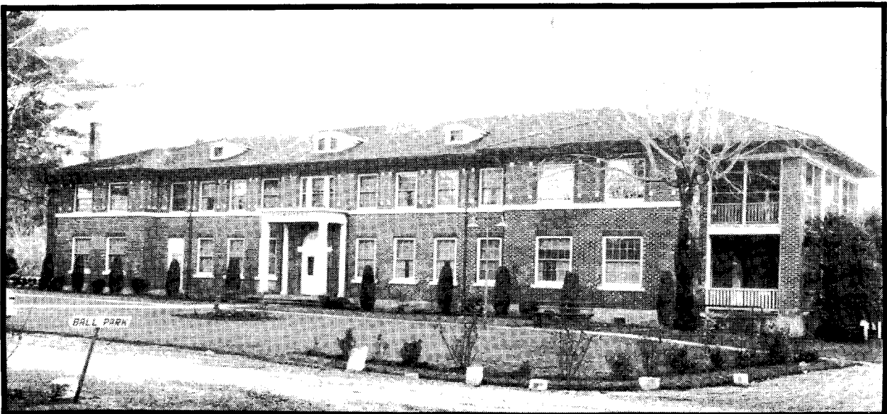
The Hospital that was damaged by the earthquake in 1965. The first floor now houses Administrative Services.
